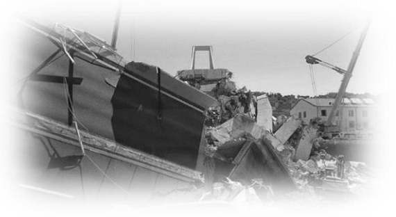
MORANDI BRIDGE COLLAPSE AUGUST 14th, 2018
