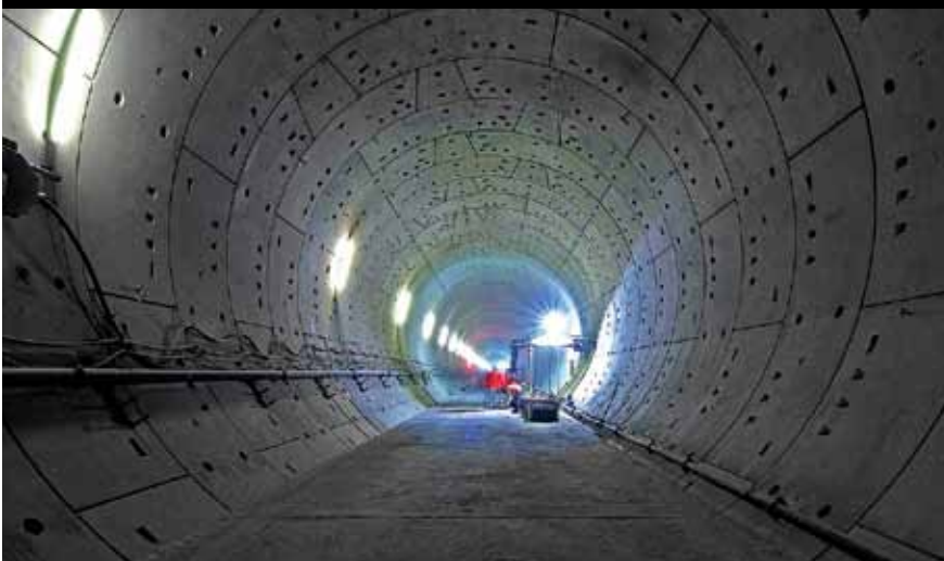
EnDurCrete will be tested in demanding environments, including tunnels
