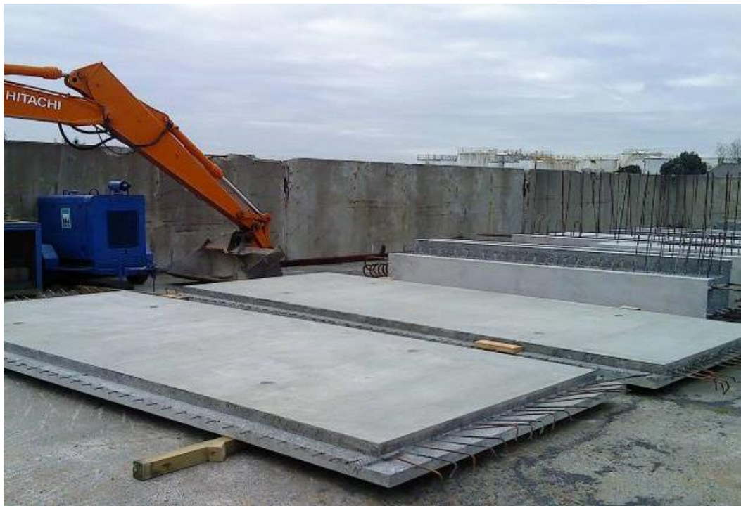
Figure 6: Precast reinforced solid slabs for wharf construction.
