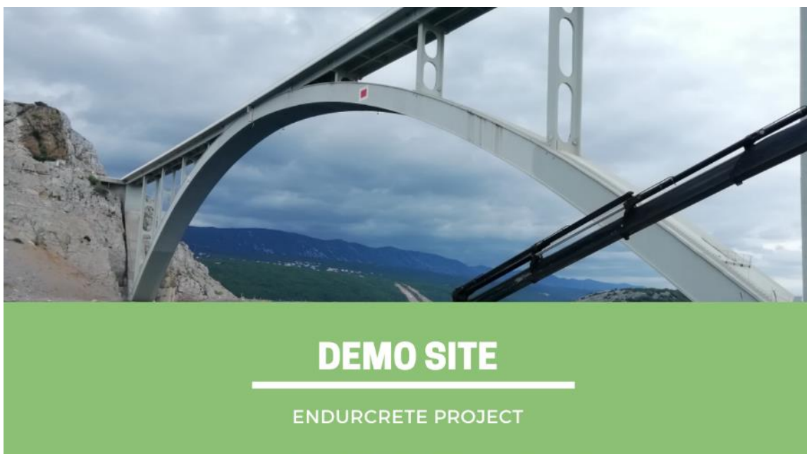
Figure 10: Thumbnail of the video 'Demo site Krk bridge'
