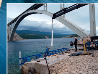
Installation of the EnDurCrete technologies at the Krk Bridge in Croatia.
